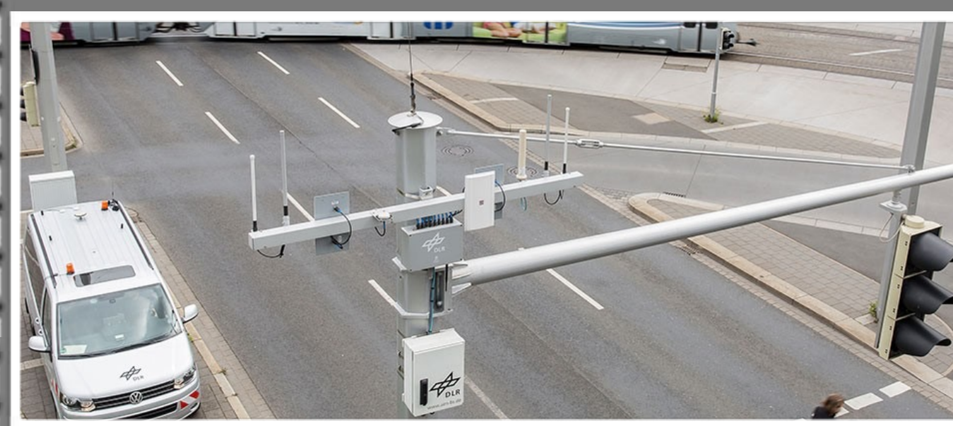
Figure 2: Smart traffic lighth for ambulance. Source: Smart Traffic Light , 2015. [8].
